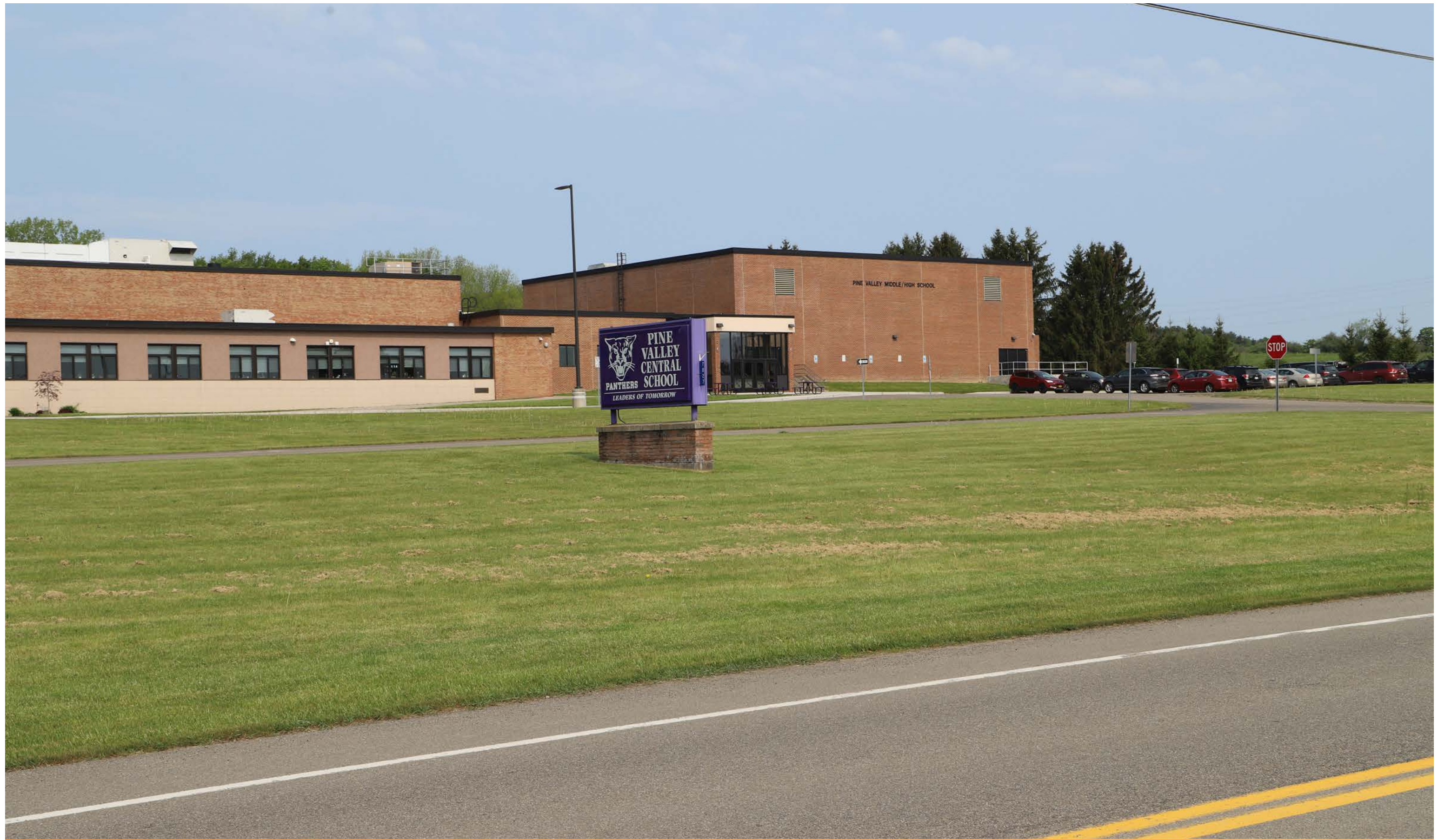
Photo 1 - NY83 at Pine Valley Central School EXISTING CONDITION
