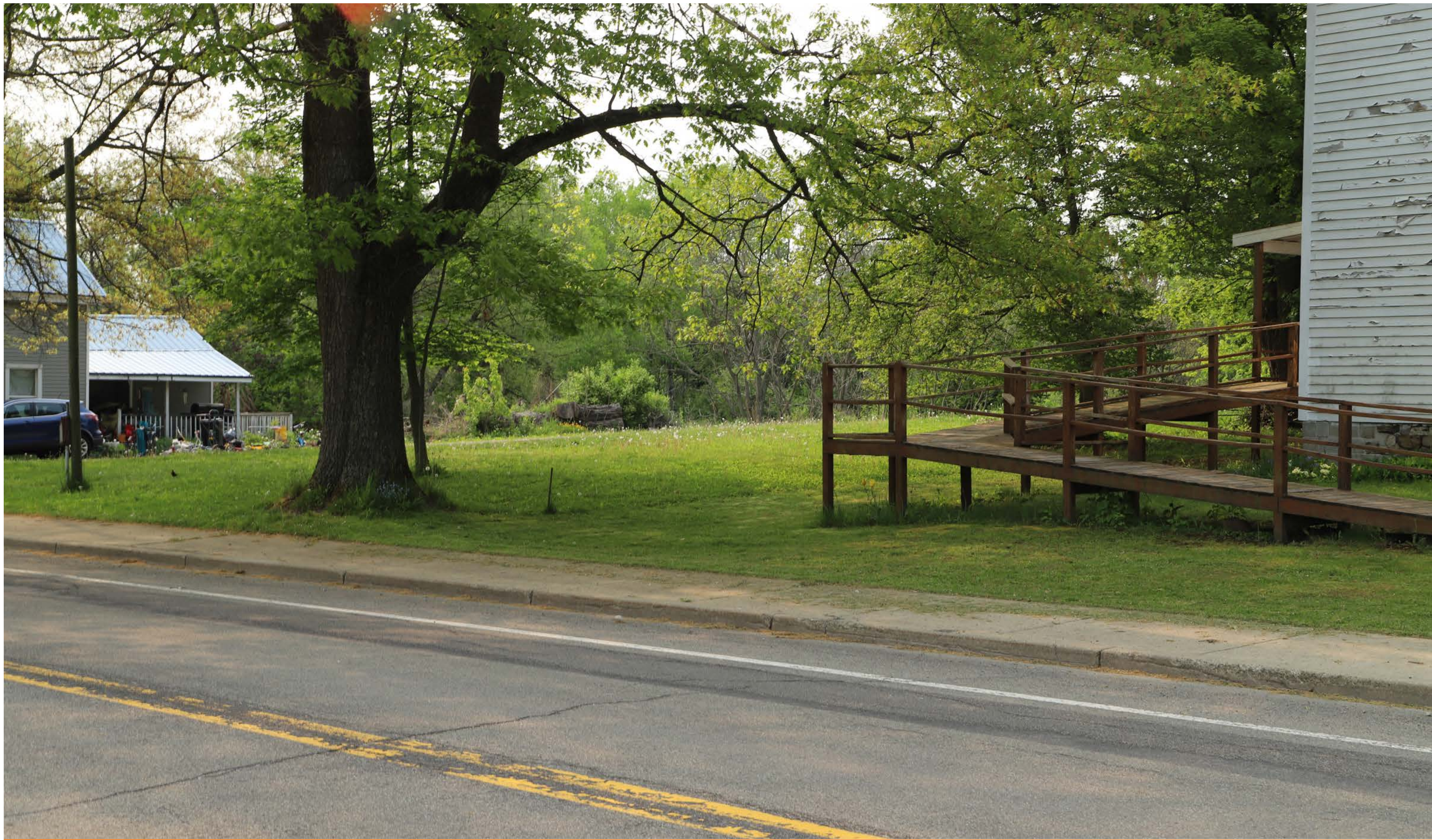
Photo 4 - NY83 at Hamlet United Methodist Church EXISTING CONDITION
