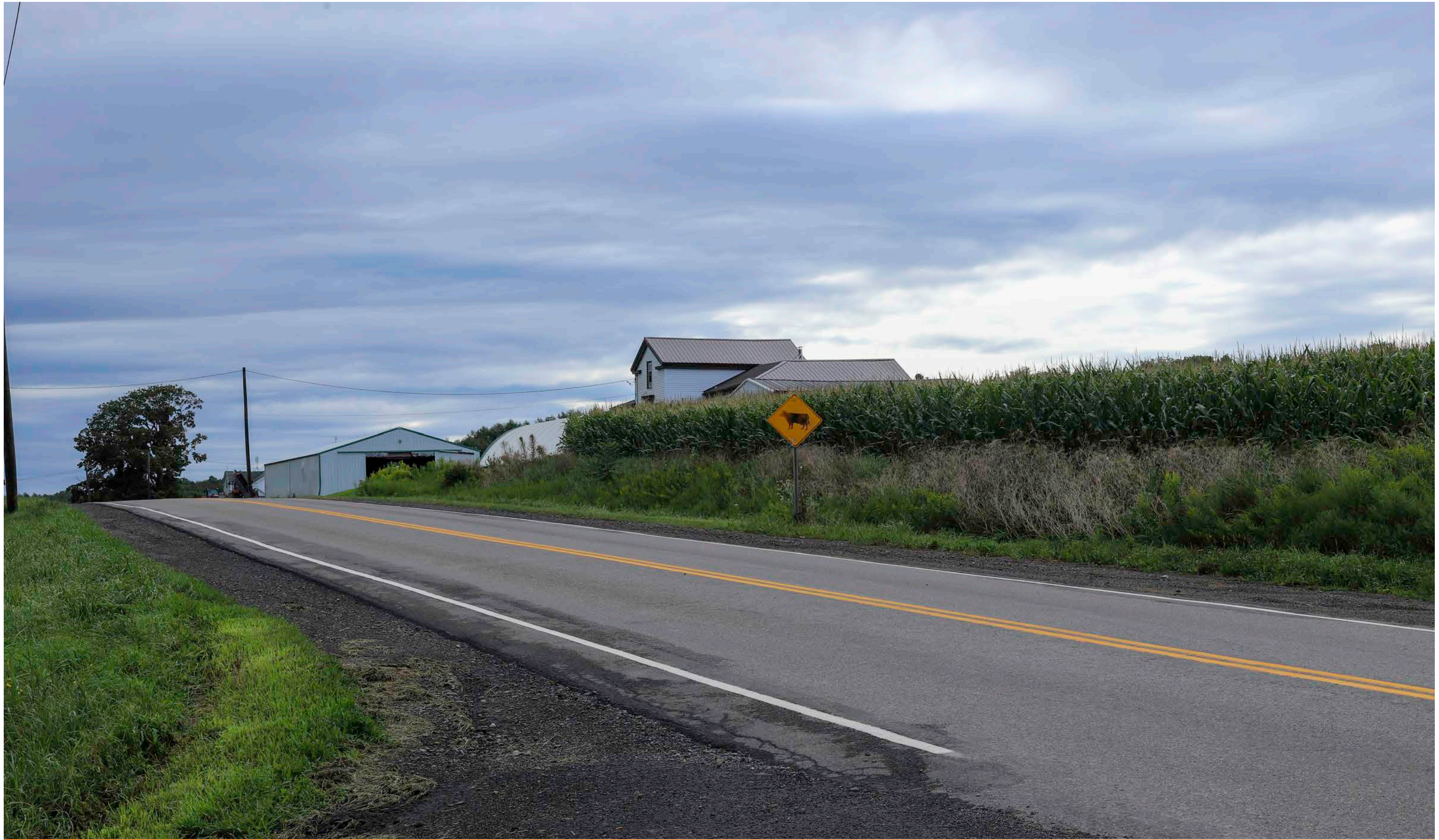
Photo 6 - Wentworth Road at Cassadaga Road EXISTING CONDITION
